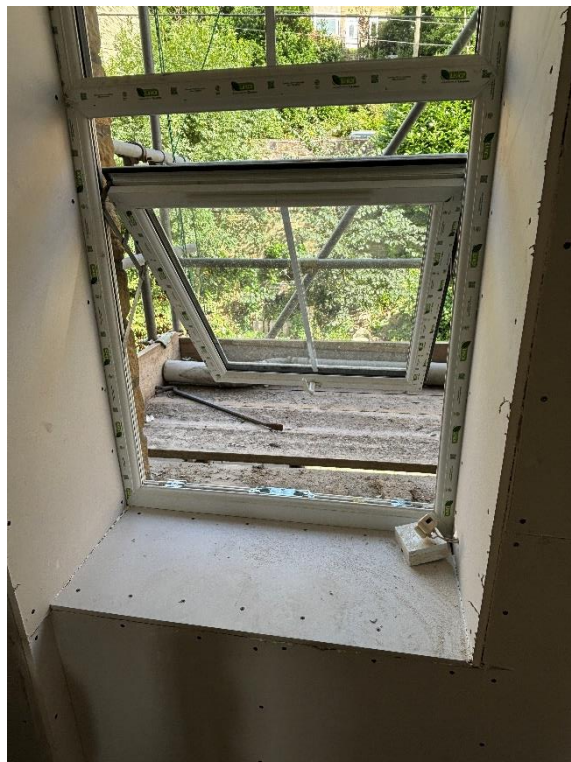
2. Fire escape window at first floor landing
