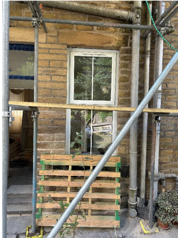
1. Window replacement has commenced
