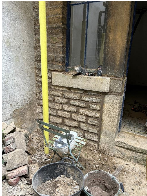
8. Repointing work to the rear elevation.
