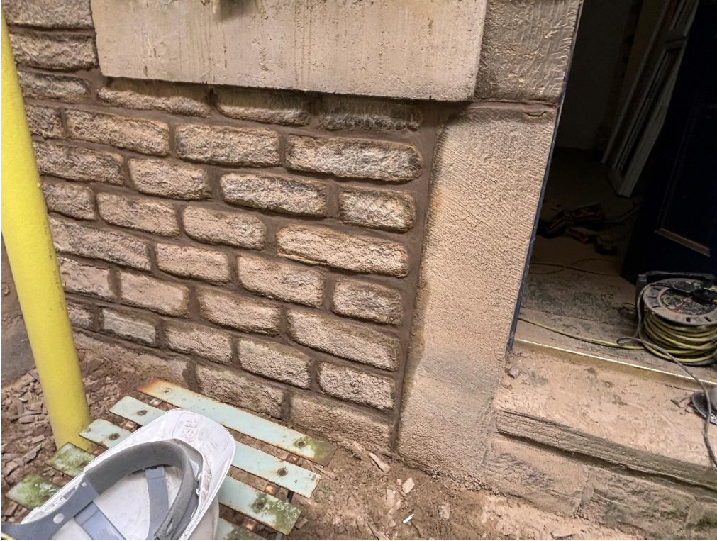
9. Repointing using a lime based mortar.
