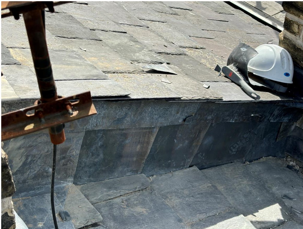
4. Additional lead flashing to the West elevation.
