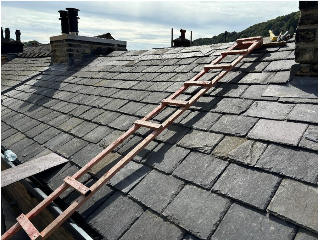
5. Roof is re-tiled and chimney stacks re-pointed.
