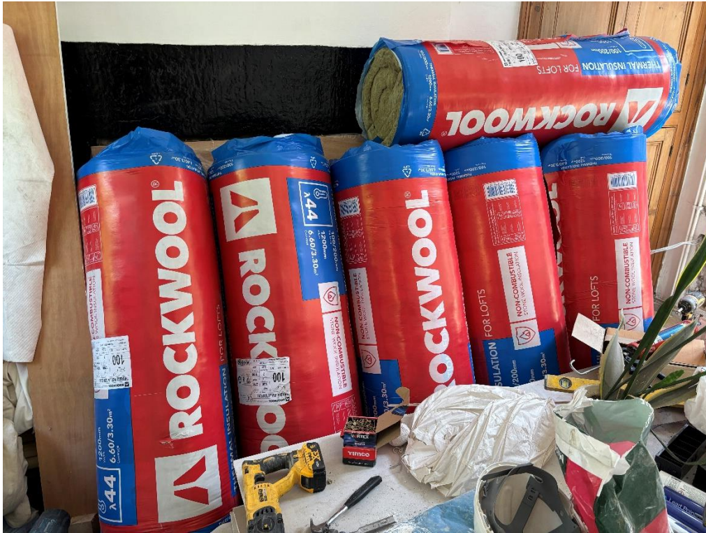
7. Evidence of Rockwool breathable insulation.
